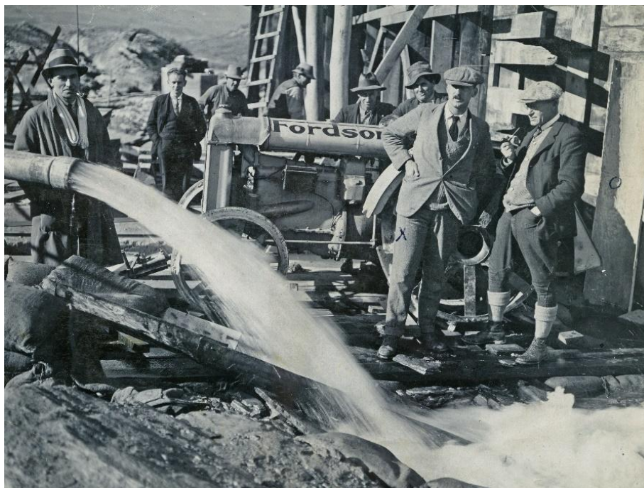
A Fordson tractor pumping out No 4 pier site ( LDM EL6517 )
