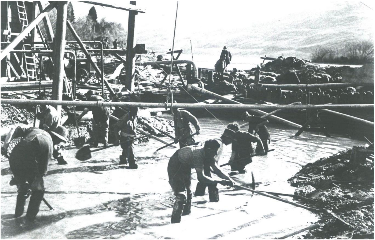
Excavating the base of a pier with picks and shovels, October 1925 (Hocken Snapshot)
