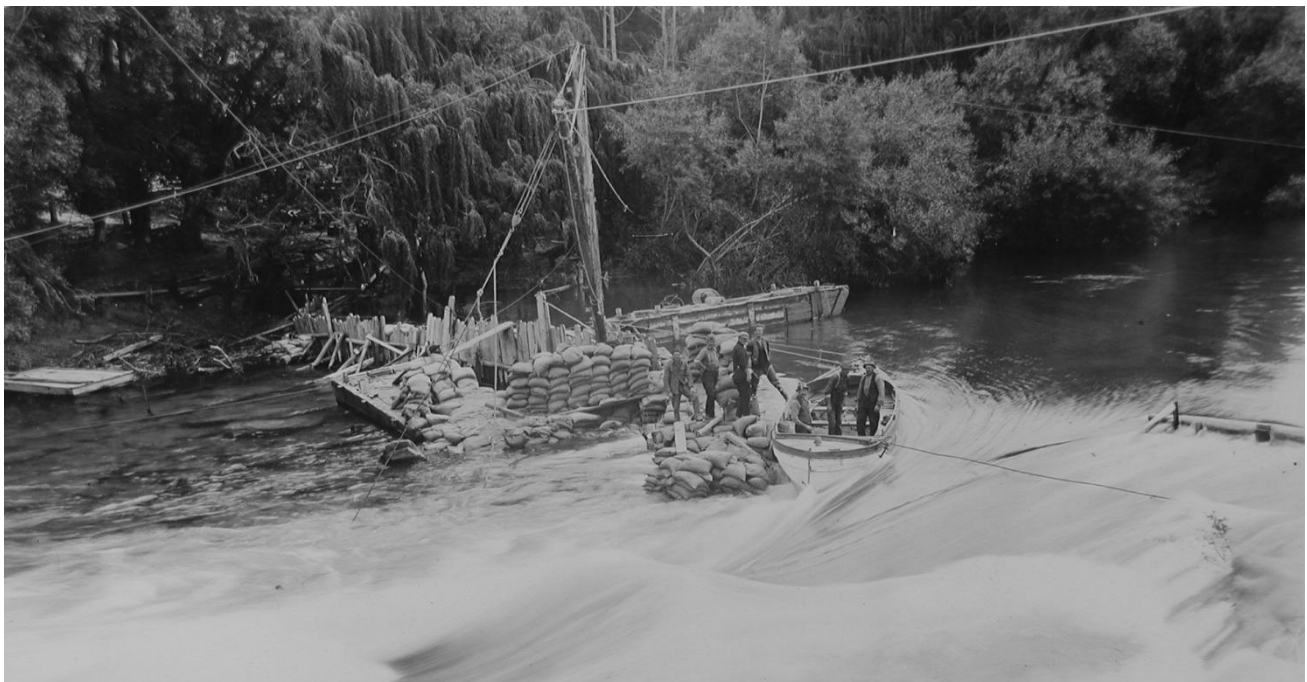
A wing dam being built at the site of No 10 pier beside the south bank ( LDM EL6720 )
